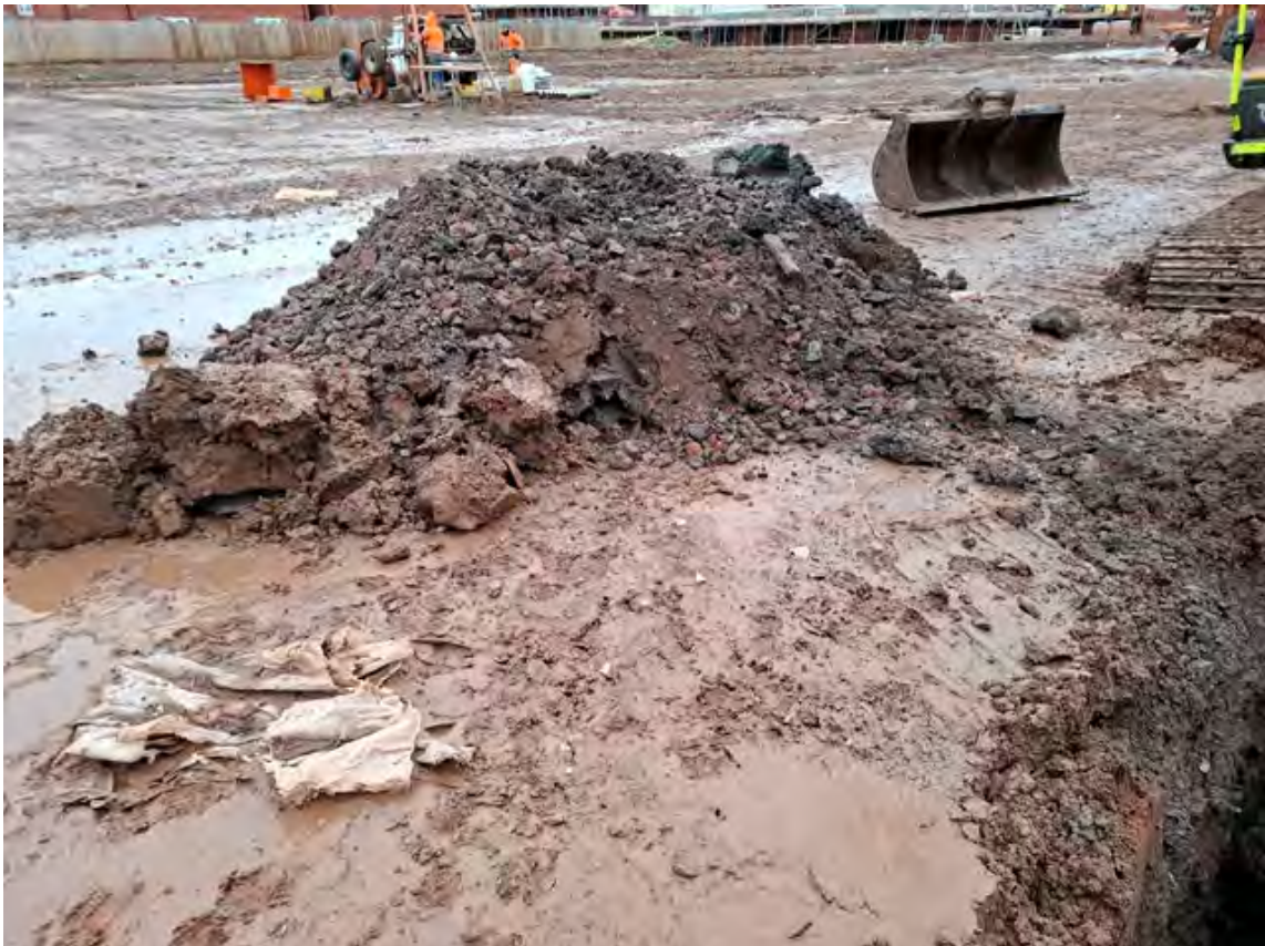
Trial Pit TP05 – Made Ground arisings
