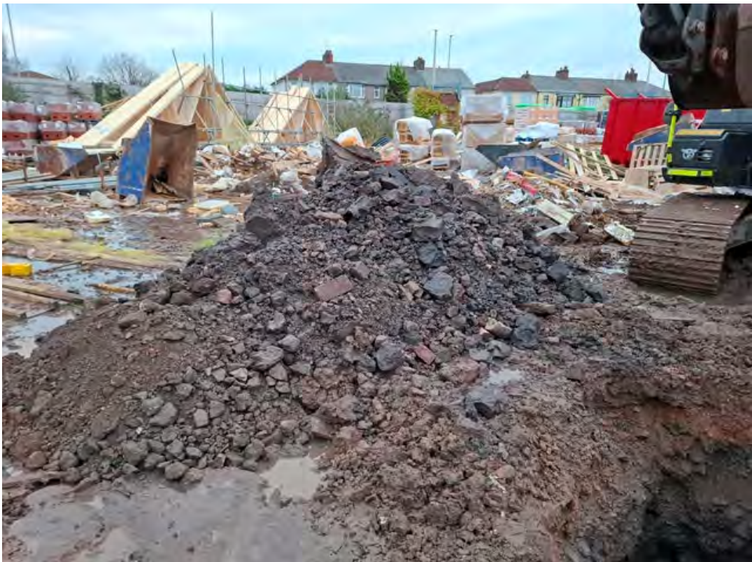
Trial Pit TP01 – Made Ground arising
