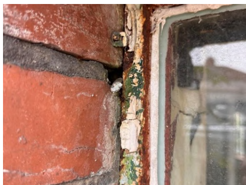
Photograph 6: u1b5-2 Missing mortar (external).
