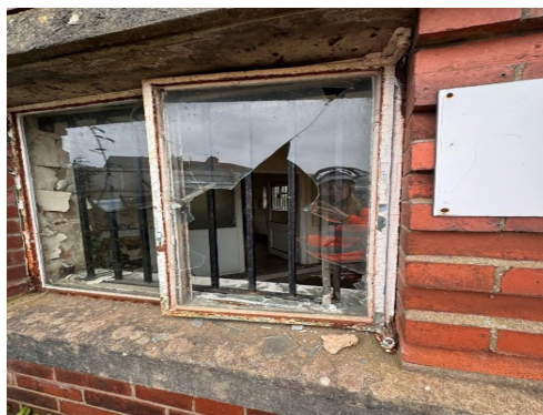
Photograph 4: u1b5-2 Broken window as an access point.
