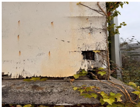
Photograph 2: u1b5-1 Hole in the window boarding.
