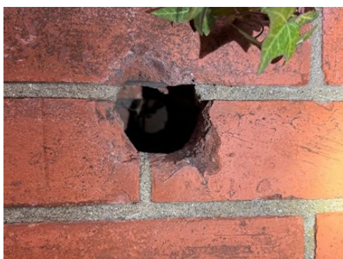
Photograph 7: u1b5-2 Hole in the brick work into cavity wall.
